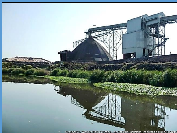
Winsford Rock Salt Mine in Cheshire. The southern end of the covered conveyor, where salt is tipped into a domed store
