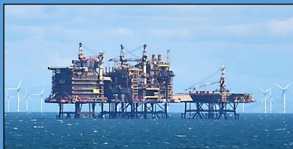
The Central Processing Platform, a three-platform, bridge-linked complex with a flare boom tower
