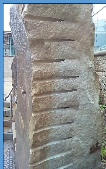
Carboniferous sandstone block, split away from the face by the plug and feather method (two metal wedges are forced apart by hammering in a third wedge, the plug).
