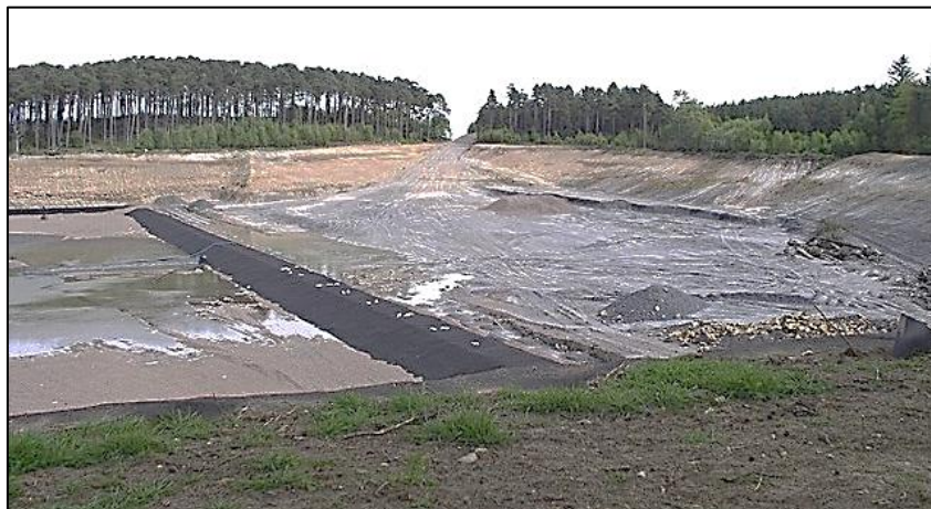
Figure 6.10. Laying black membrane as part of landfill site preparation, Drummond Moor, Howgate, Midlothian, Scotland
