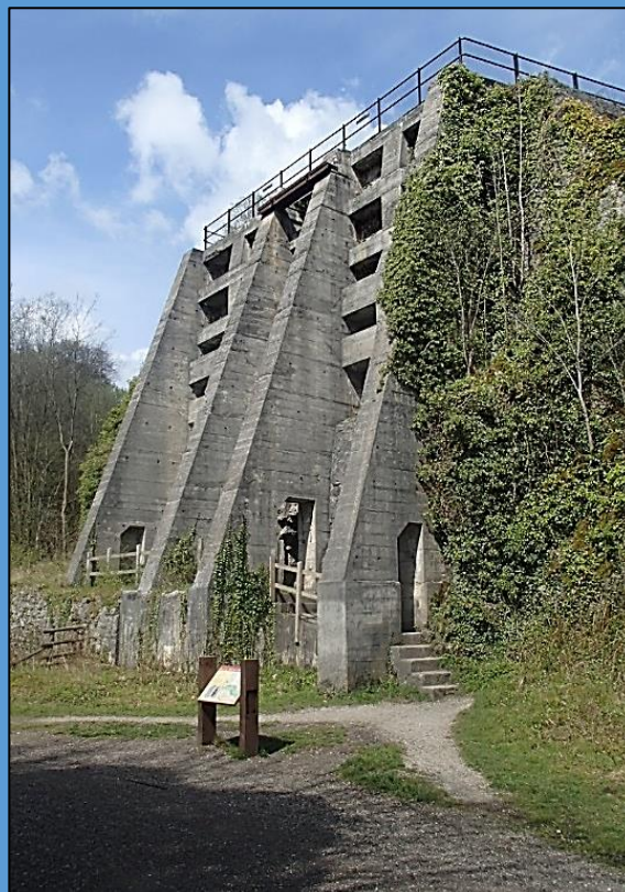
An industrial scale limekiln beside the former mainline railway near Millers Dale, Derbyshire. The kiln built in 1880 was closed in 1944. It produced 50 tonnes of quicklime per day
