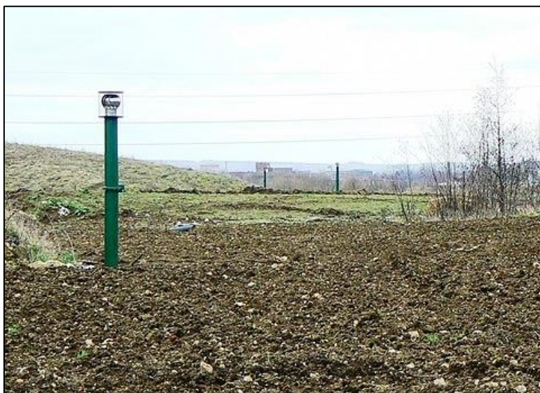
Figure 6.11. Methane gas vents on an old landfill site, Shaw Forest Park, Swindon, Wiltshire
