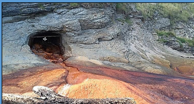
Iron oxide-polluted water flowing from an old mine tunnel, Spittal, Northumberland in northern England
