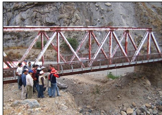
Field School in Matucana high risk sector: beside debris flow (2010).
