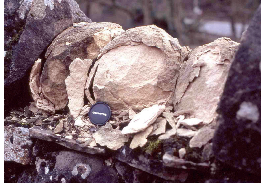
The effects of freeze/thaw weathering in a porous limestone (Photo: Peter Kennett )
