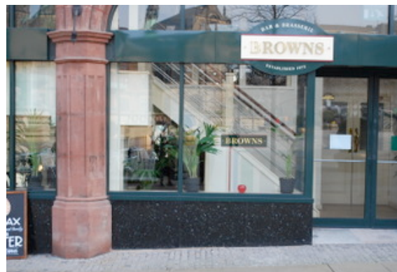
Building stones in a city centre – red sandstone and ‘granite’ make up the front of the café, whilst granites and buff sandstones form the paving. St Paul’s Parade, Sheffield (Photo: Peter Kennett)
