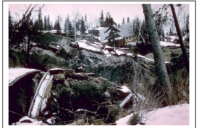
Buildings carried by a landslide - the Turnagain Heights landslide in Anchorage. 75 homes slumped, twisted, or collapsed when liquefaction of subsoils caused parts of the suburban area to move up to 700 metres during the 1964 earthquake (9.2 magnitude).
